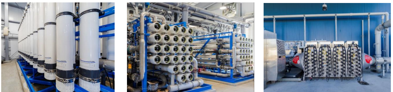
Figure 8: Pure Water Soquel Treatment Steps including ultra filtration membranes, reverse osmosis, and ultraviolet light.
