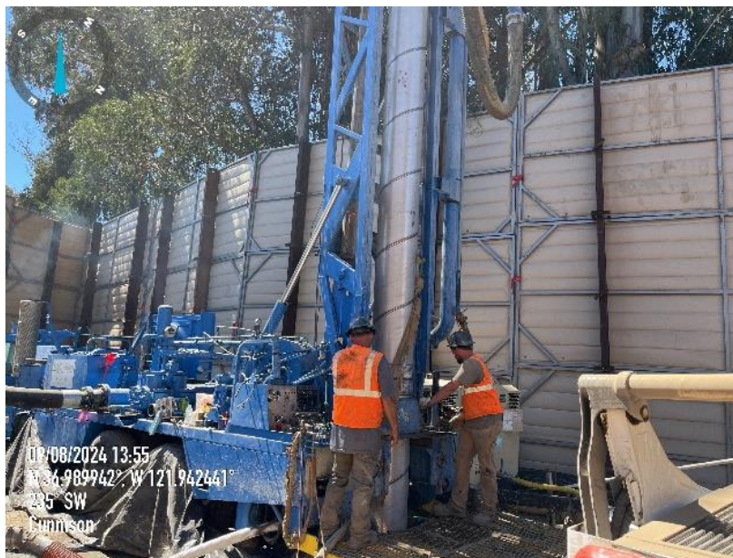
Figure 6: Cunnison Well drilling. Photo courtesy of SqCWD.
