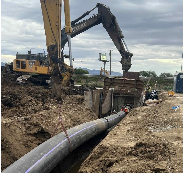
Figure 8: Pipe for the College Lake Project. Source: PV Water.
