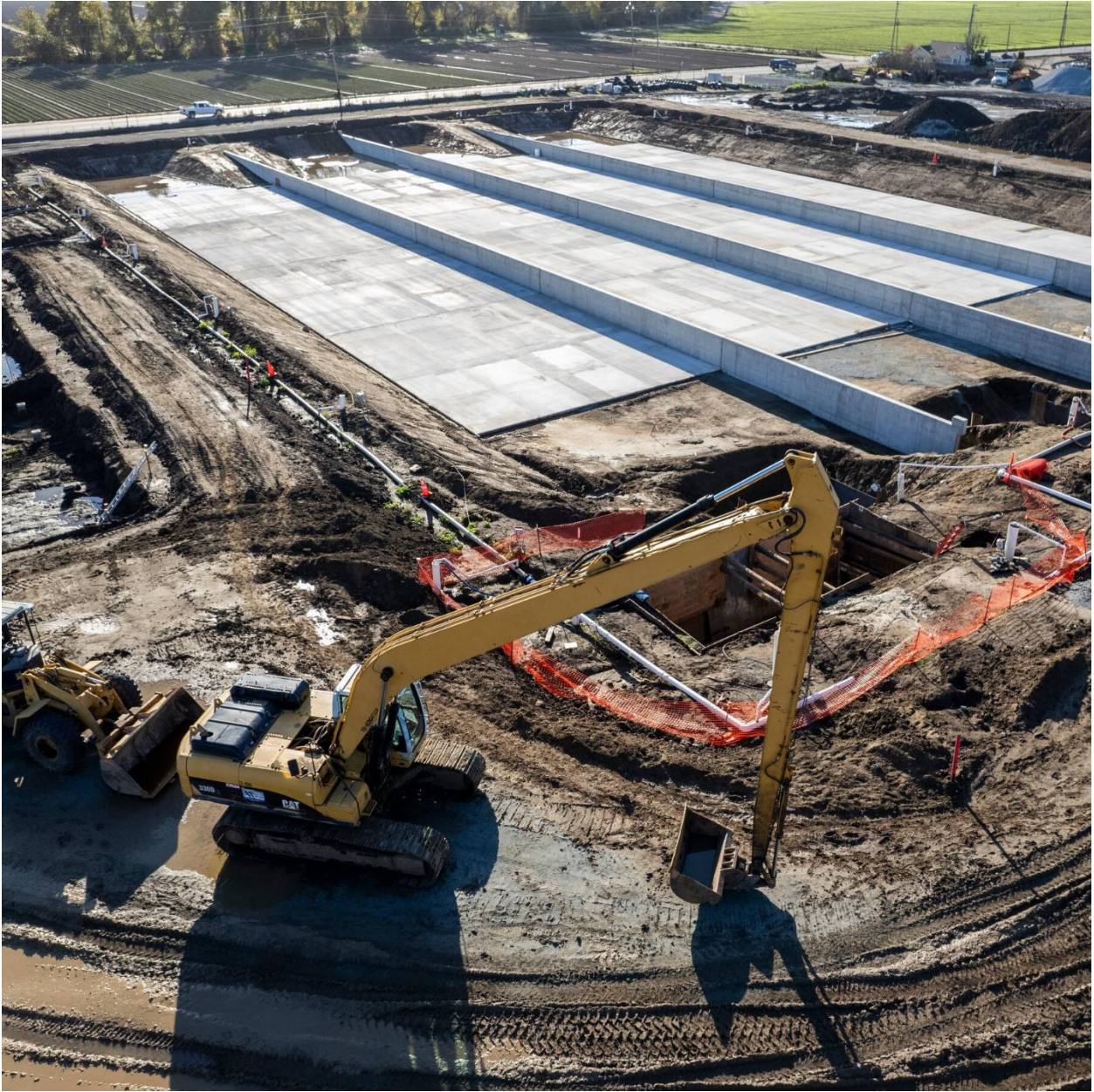
A new reservoir to capture rainwater.
