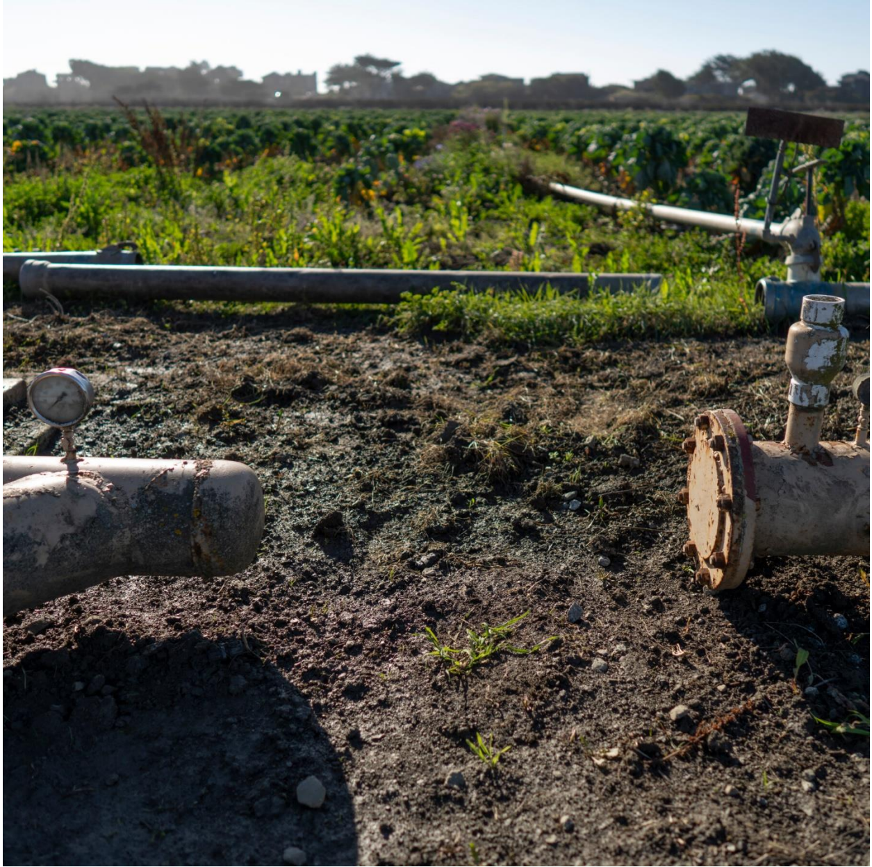
A well pipe capped years ago to stop saltwater intrusion.
