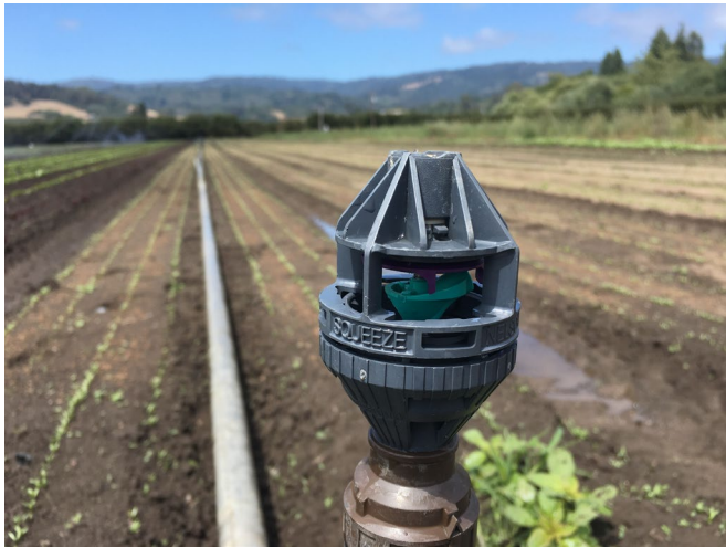
Efficient sprinkler heads
