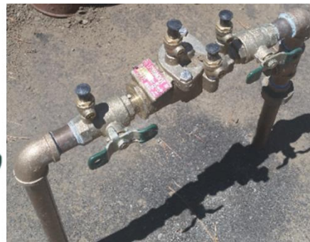
Fig. 2 - a reduced pressure principle backflow prevention assembly
